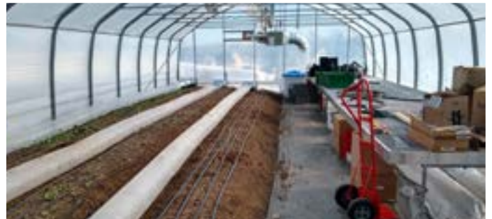
The interior of a greenhouse features a positive-pressure air core heating system. (© CISA, 2022)
